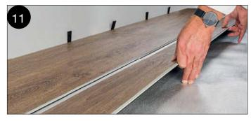
DISASSEMBLING THE LONG SIDE Lift up the entire row in the same angle as you did during installation, then slide the rows apart.
