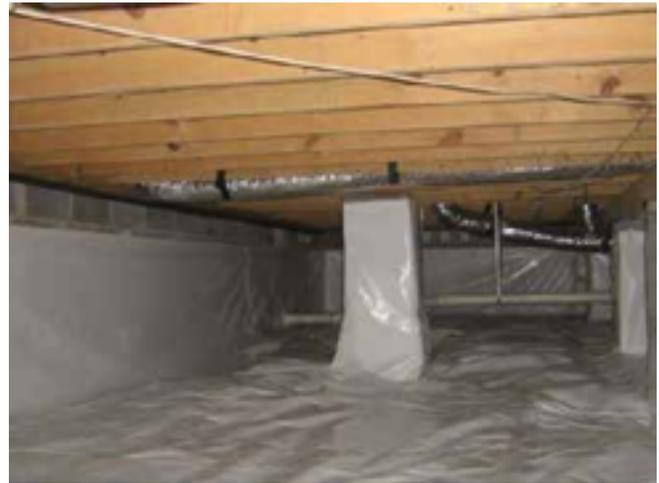
(no exterior cross-ventilation) require a dehumidification system as part of the sealed crawlspace design.
